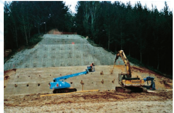
(Above) Screw pile installation, showing benching
