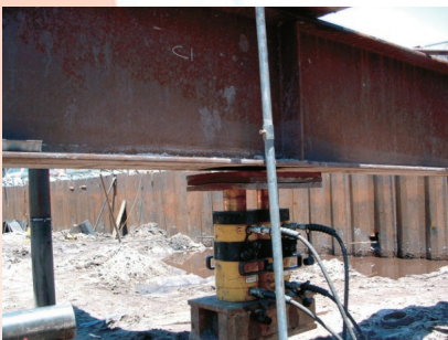
(left) Proof loading the screw piles to ensure that the design capacity is reached
