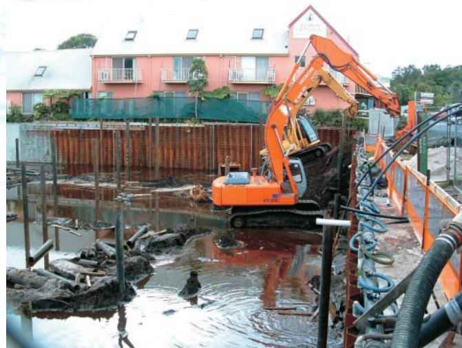
(above) Sheet piling in place, with shotcreting evident at rear left, screw pile installation in progress
