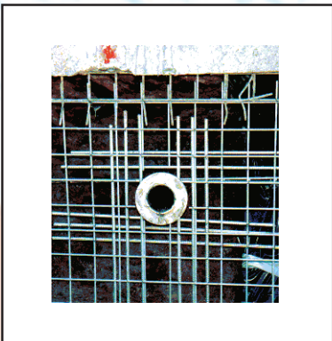
(left) Flange welded to the pile cap to allow tensioning
